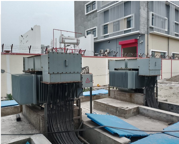
Transformer S11-3000kVA-11/0.415kV
