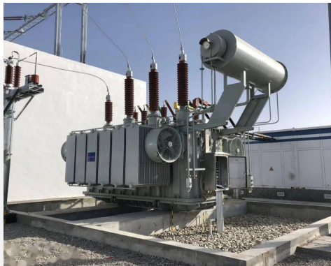
Transformer SFZ-10MVA-110/10
